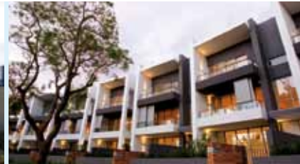
THE PENINSULA, BURSWOOD, WA
