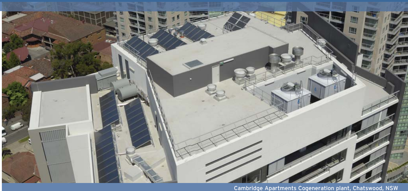
Cambridge Apartments Cogeneration plant, Chatswood, NSW
