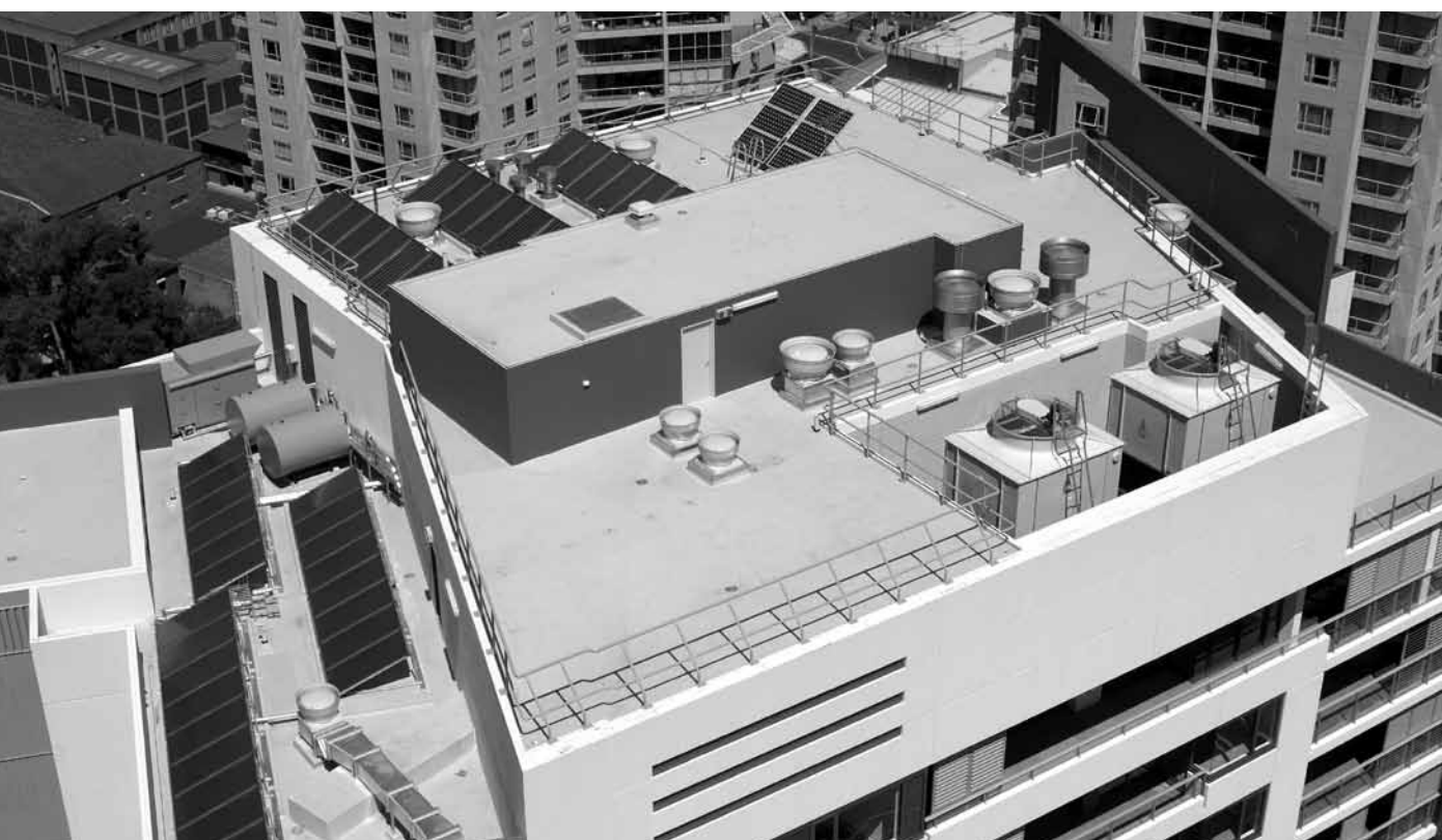
Cambridge Apartments cogeneration plant, Chatswood, NSW
