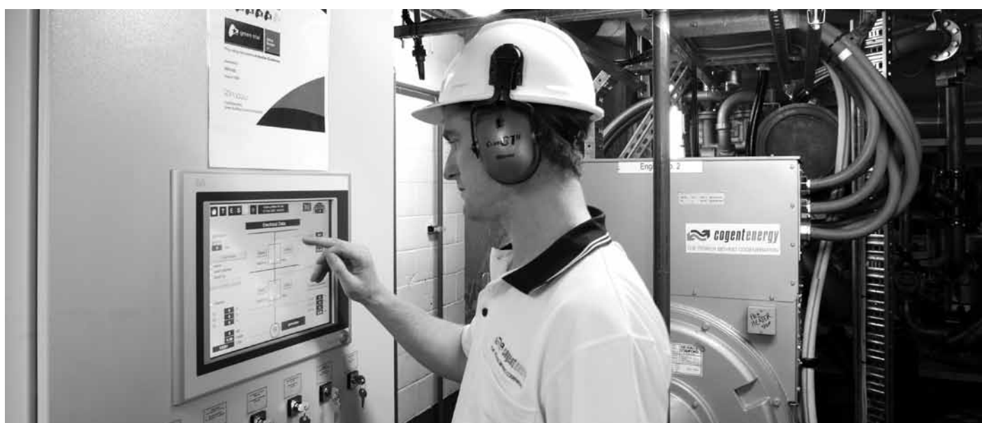
101 Miller Street North Sydney plant room, NSW
