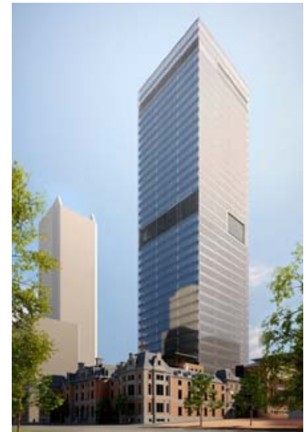
OLD TREASURY BUILDING, WA
