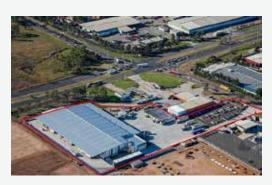
8 Brabham Drive is an A-grade industrial logistics facility designed as a cross-dock incorporating a high-clearance, column-free warehouse. On a long-term lease to specialist logistics operator BagTrans, it also features over one hectare of heavy-duty, concrete hard stand areas, as well as a truck-washing facility.
